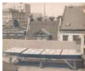
First ever solar panels installed
